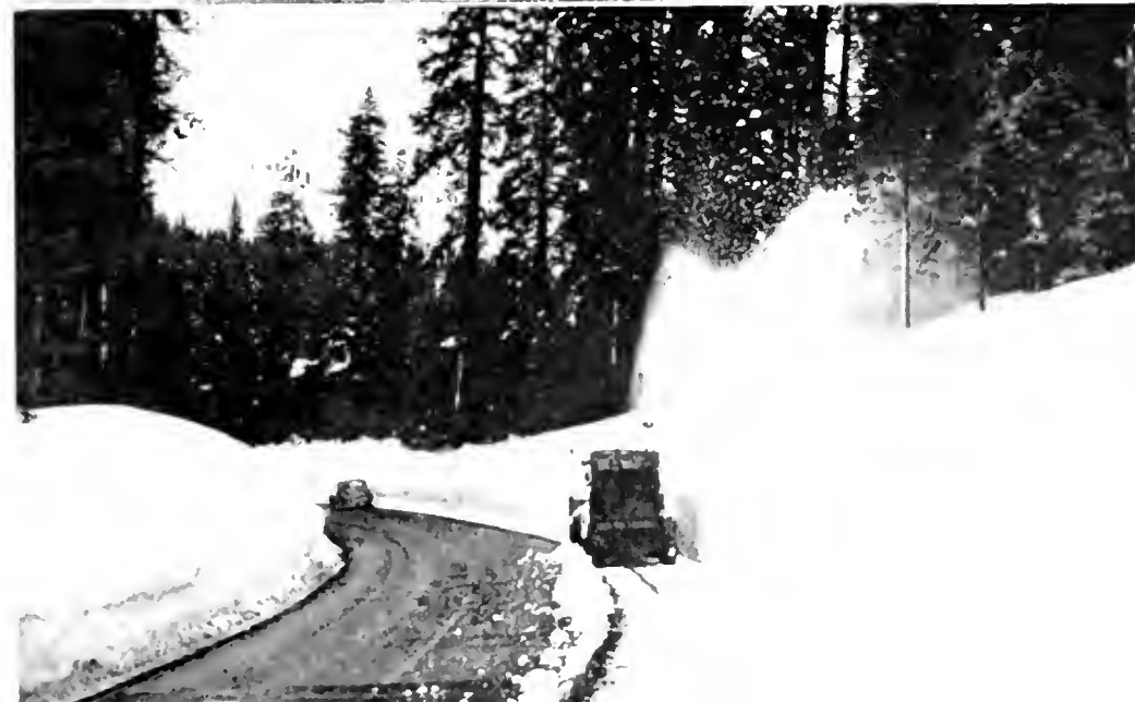
Push plows of several types shown in the two upper photos aided by a rotary plow kept State Highway 36, the Red Bluff-Susanville lateral, open during an 8-foot snowfall on March 3d to 5th
